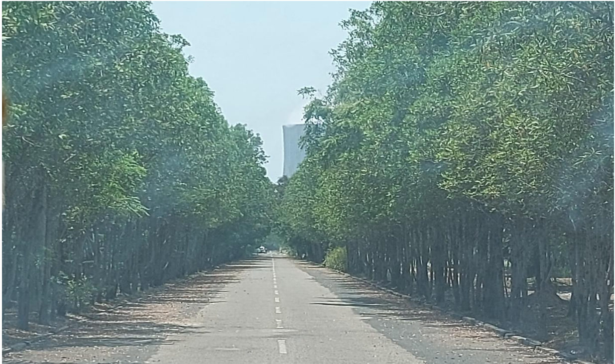
GREEN COVER ALONG PIPE RACK & INTERNAL ROADS
